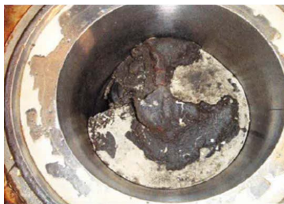
Figure 1: Illustration of salt build-up and blockages in topsides gas flowlines and processing equipment. Images courtesy of Perenco UK.
