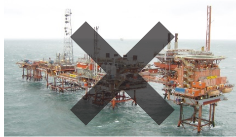
Decommission 27A Compression
