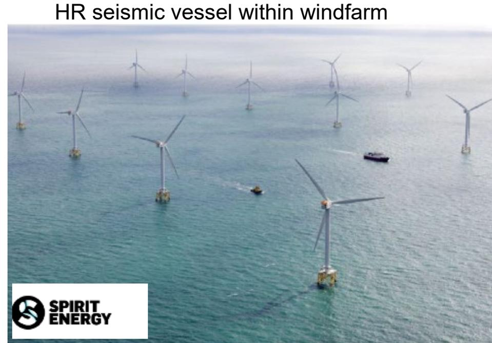
A 2DHR seismic survey was acquired over Knox and Lowry in Q1 2013 included shooting through the Ormonde windfarm – a UK first. Extensive planning and pre-survey modelling were required.
